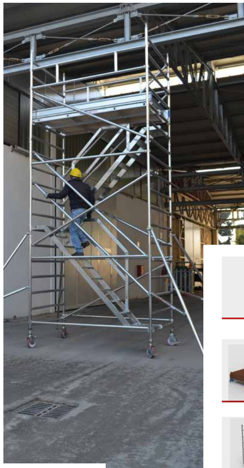
CONFIGURAZIONE CON SCALA A RAMPA ALTERNATE E CONTINUE Configuration with alternating continuous ramp ladders
